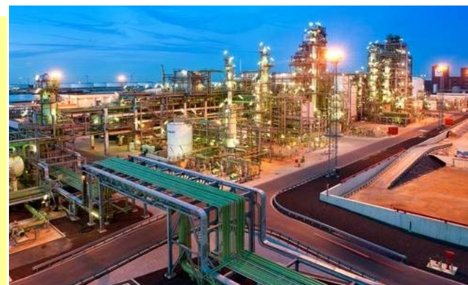
Rotterdam Next BTL plant started up Sept. 2011.
